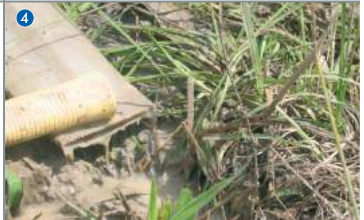
Drive Plati-Drain® into optimum position
